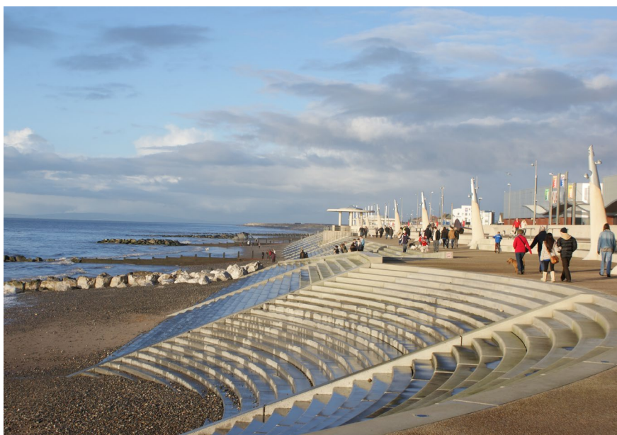
Cleveleys Coastal Protection Scheme, UK. Source: Wyre Council
