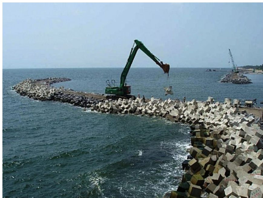
Construction of a dam. Source: DMC.
