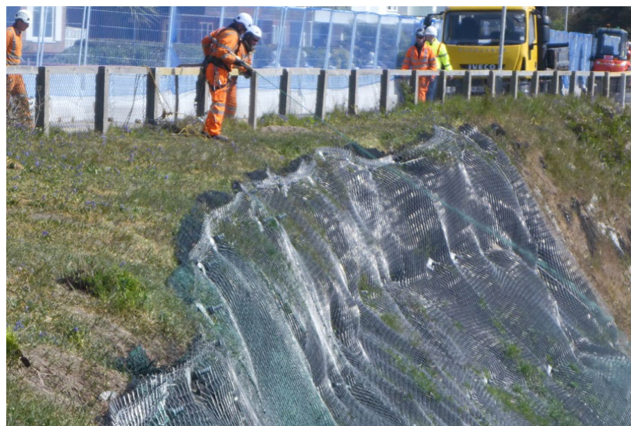
Stabilisation work at Canford Cliffs, UK . Source: BCP Council.
