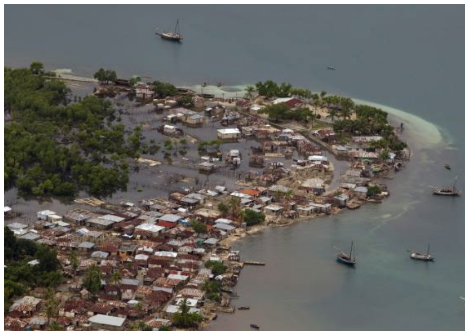
Coastal flooding episode. Source: Logan Abassi.
