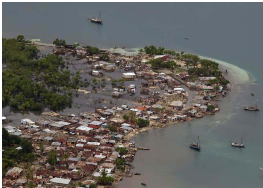
Coastal flooding episode. Source: Logan Abassi..
