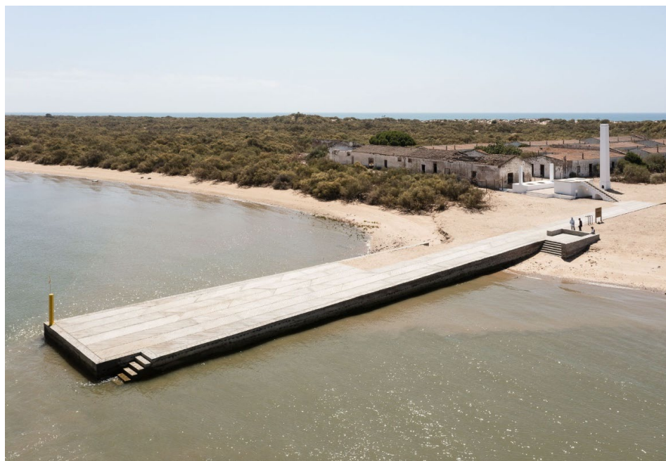
Groynes at the Alambra del Rompido, Spain. Source: Sol89 Architects.
